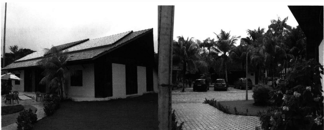
Figure 8: Farm Hotel Paraíso in Mosqueiro
